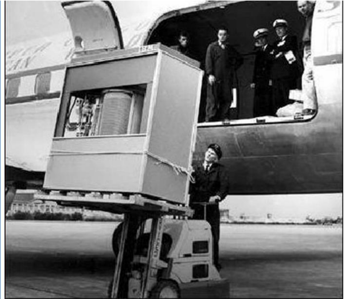
This is a picture of IBM 350, the first hard disk in history with storage capacity of nearly 5 MB
